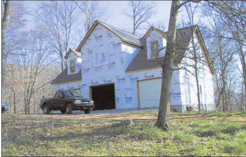
A Tyvek house wrap is one way of helping stop the air infiltration in your new home. Caulking, insulation and efficient windows are also important in reducing air leaks.
