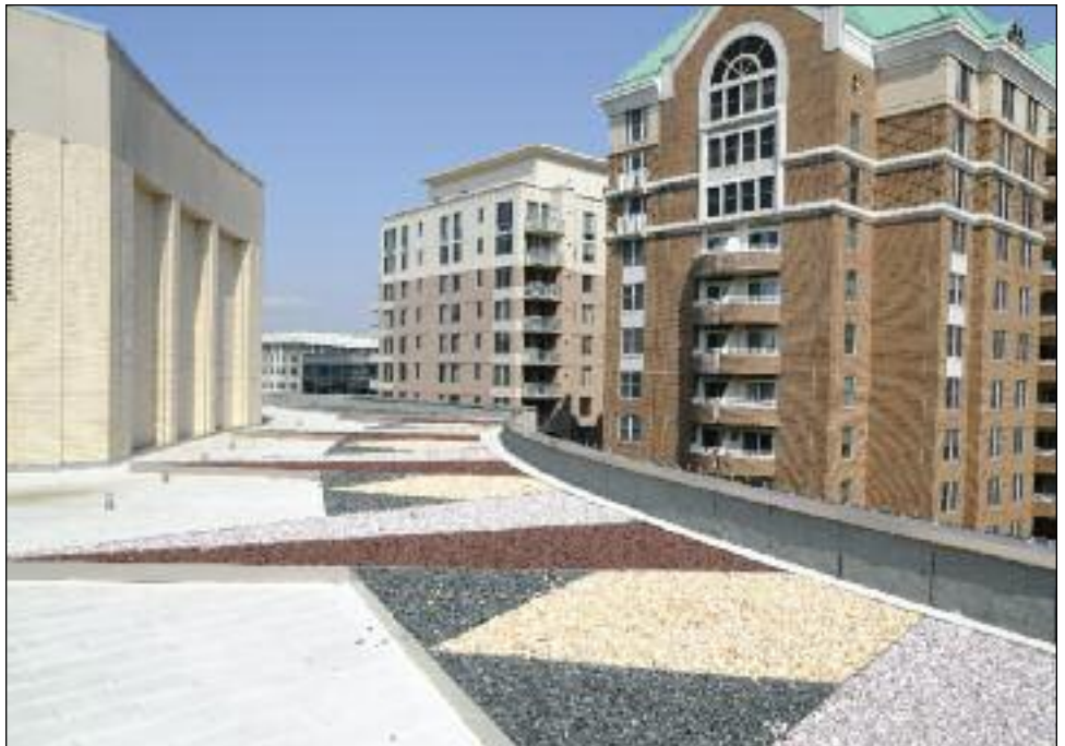
Light-colored, heat-reflective tiles cover the roof of the NRECA headquarters building in Arlington, Va., reducing the urban heat island effect. Photo by Michael Lynch, NRECA
