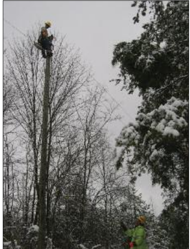
Restoring power after a heavy, wet snow is a time-consuming process. Foreman Leonard Eidson and his line crew had to cut several trees and clear the road just to get to this outage location. After hiking up the hill to get to the downed line at left, the Holston EC crew had to pull the cable out of fallen trees and brush so they could splice the line together. Above, Jarrod Bachman, on the pole, and Stacy Hayes have one line span nearly repaired.
