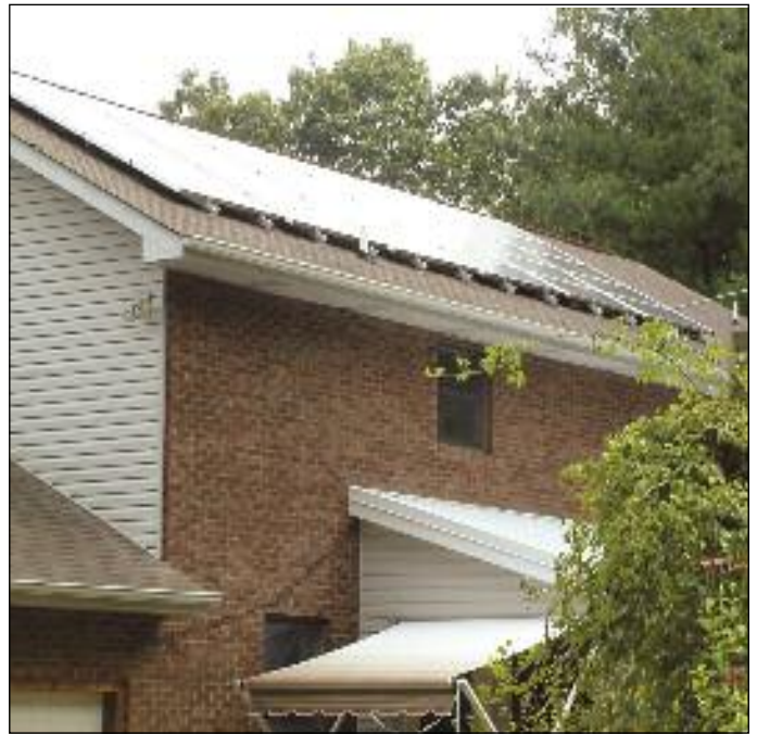
This south-facing view of the Small home shows the photovoltaic panels on the roof and the room addition that helps to cool their home in the summer and maximize thermal storage in the winter.
